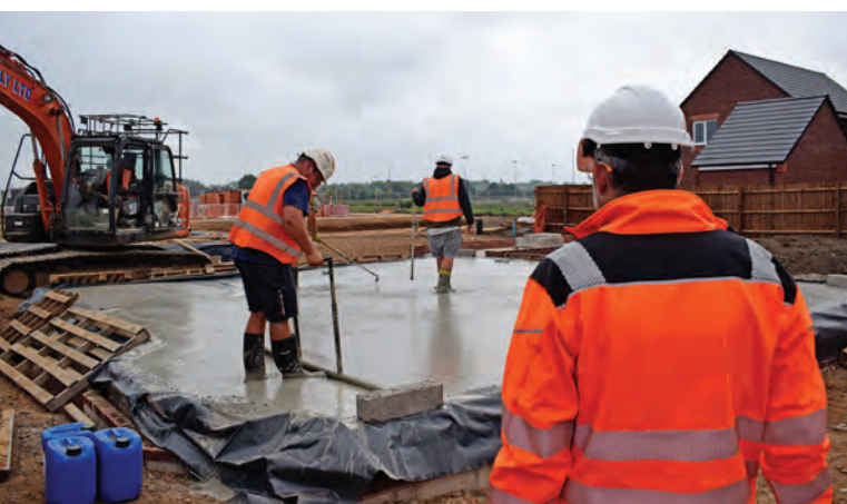
Figure 2: Level checks of the floor surface.
