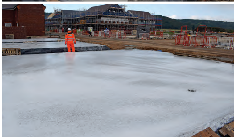
Figure 5: Curing compound applied to floor.
