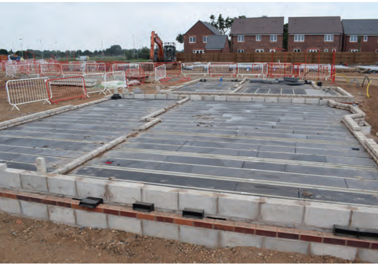
Figure 6: Beam-and-block floor system prior to membrane installation and structural concrete topping being poured.
